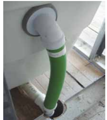
The Flex 900 Innovator® Series compensates for misalignment without installing extra fittings.
