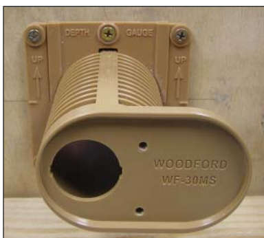
Mounting Sleeve adjusted for depth and attached to wall
