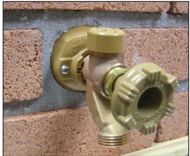
Finished brick and mortar with faucet attached to Mounting Sleeve
